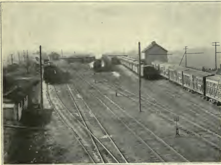
FIG. 335. FREIGHT YARDS. Argo Yard of the Indiana Harbor Belt Railroad.
